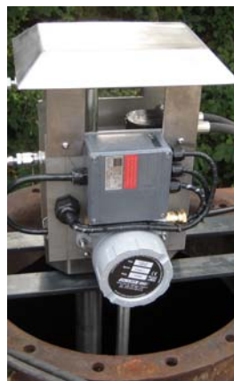
Gas detector with video camera and light
